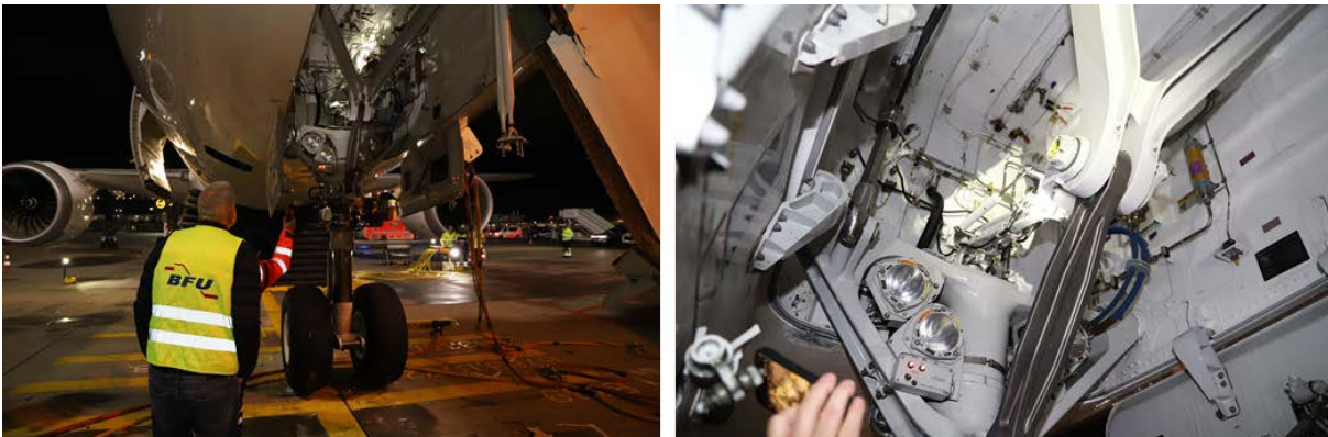
Fig. 7: Documentation of the missing landing gear downlock pin on the nose landing gear of the B787-9
